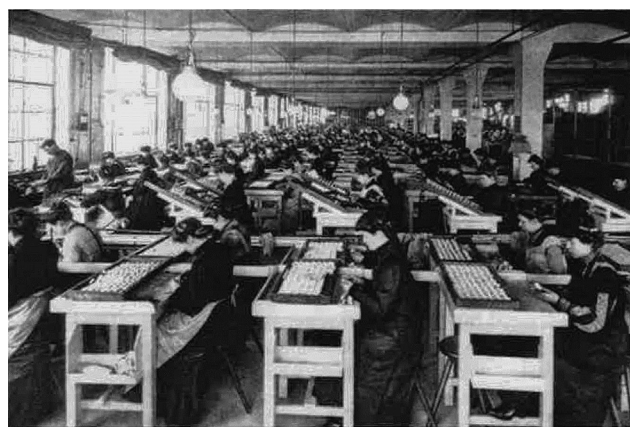
Figure 10. Fabrication of Nernst lamps around 1900 at AEG. Source: Ref. [4], p. 97.
